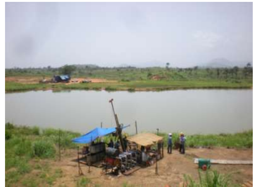
Drilling around Droujba Pipe
