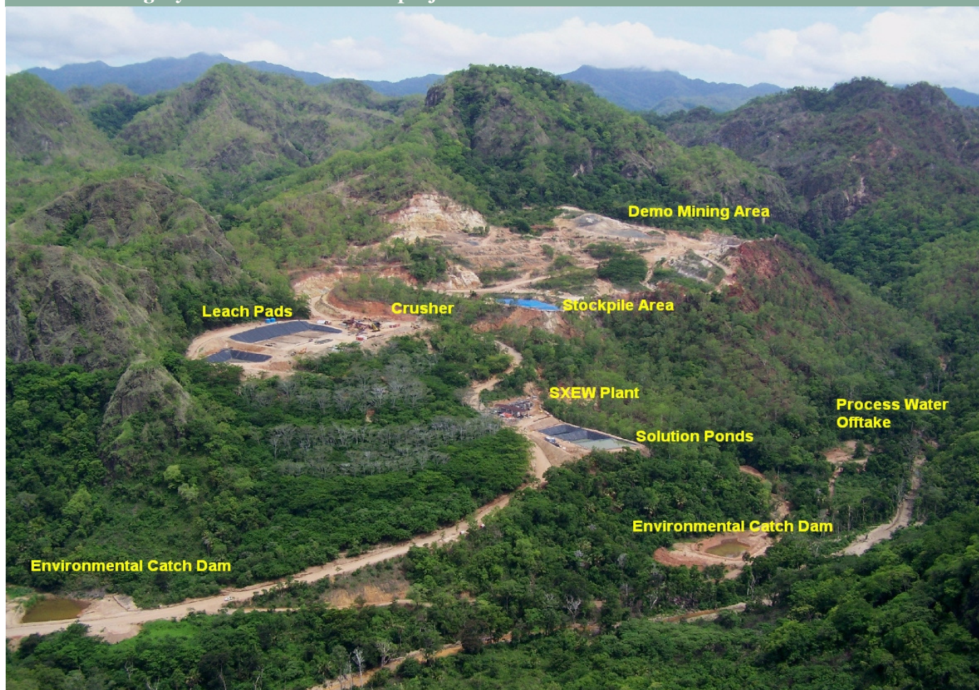
Photo showing layout of the Wetar demo project
