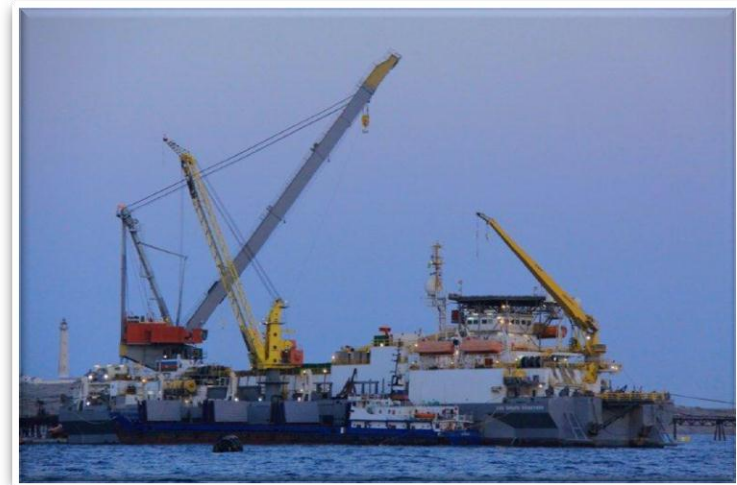
Above: Pipe-laying for the trunkline and in-field pipelines.
