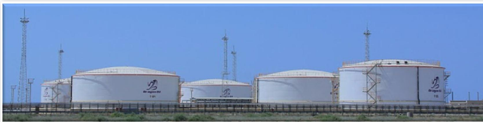
Above: Storage tankers.
