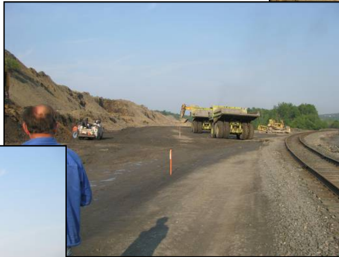
Atlantic Coal's team and equipment building the new railway embankment
