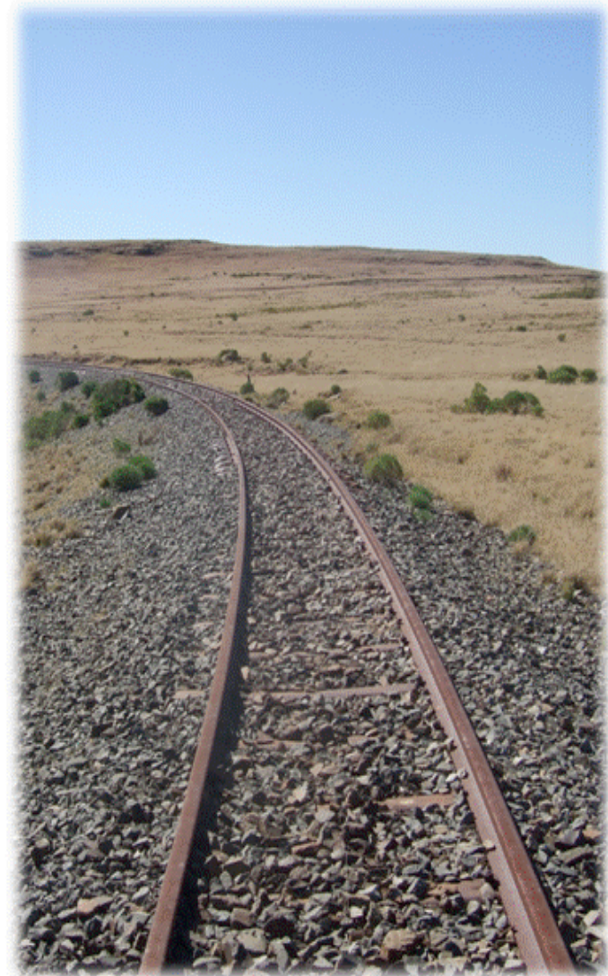
Rail Line Crossing Elitheni Rights Area
