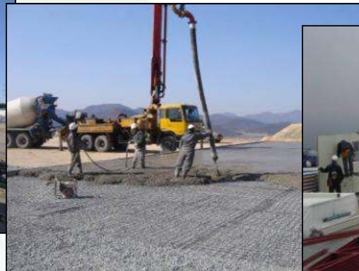
Jan 2010 Laying foundations
