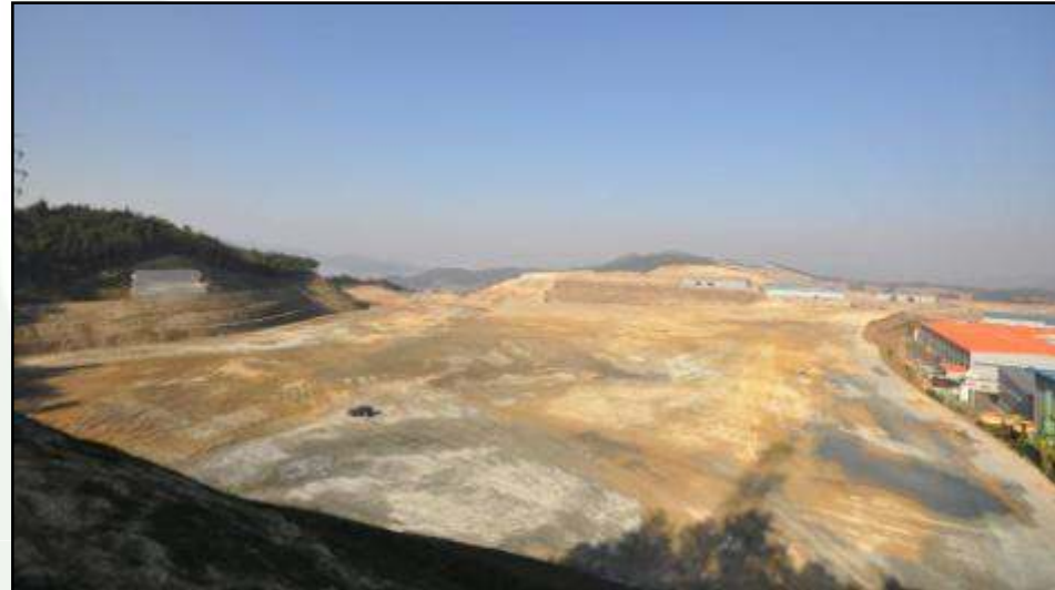
Nov 2010 Site levelled Lease signed
