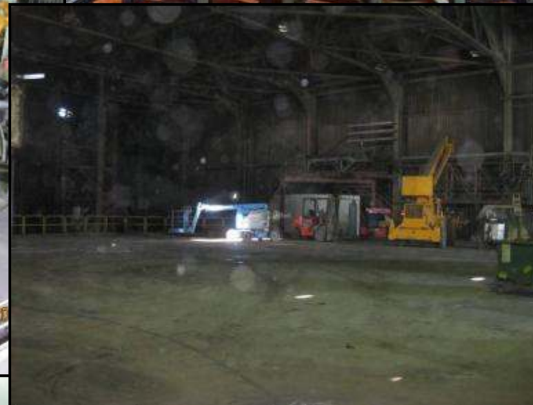
Jan 2010 Site cleared
