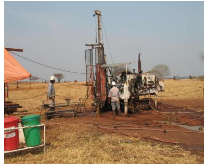
Drilling on the Araguaia project
