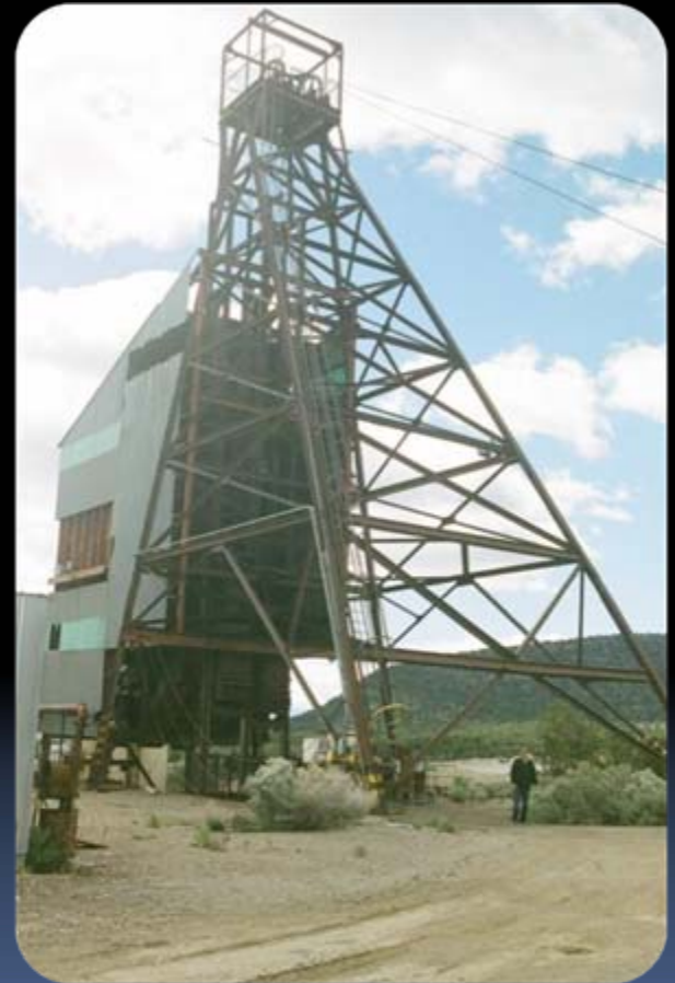
Production Shaft at Burgin Project
