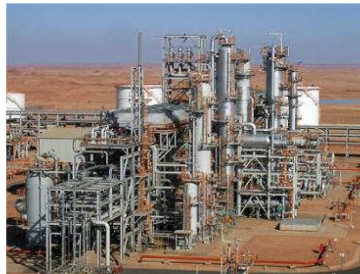
Gas Processing Plant ,TFT Field ,Illizi Basin
