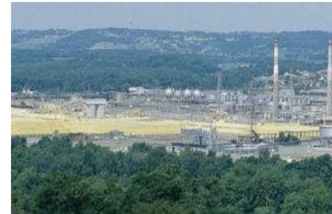
Lacq Gas Processing Facility
